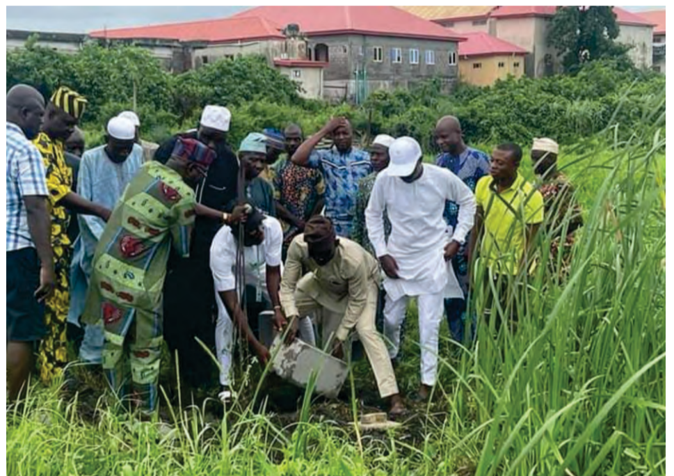
Hon. Valentine Buraimoh laying a foundation at the allocated abattoir land
